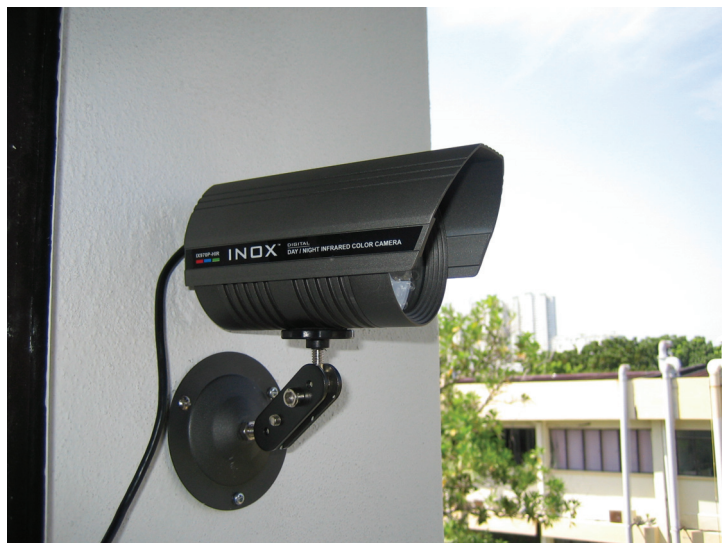
Fig. 2. Internet Video Surveillance (IVS) camera used in this study was installed at the top floor of School of Physics in Universiti Sains Malaysia.
